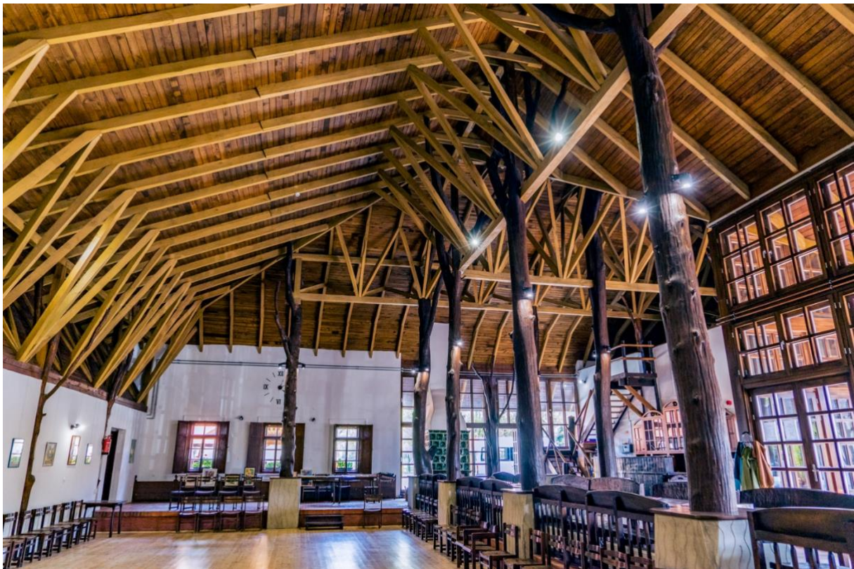
Picture 5: Village Center in Zalaszentlászló planned by Imre Makovecz (source: https://makovecz.hu/terkep/wp-content/uploads/2020/06/13706-STAT_2-1981-CONT_6-CC_HUN-KOZ-HIV-F-7.jpg Last Accessed: 30.03.2023.)
