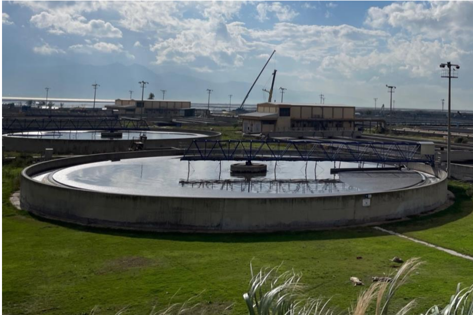
Figure 7: Çiğli Wastewater Treatment Plant, behind Çiğli Wetland. 141
