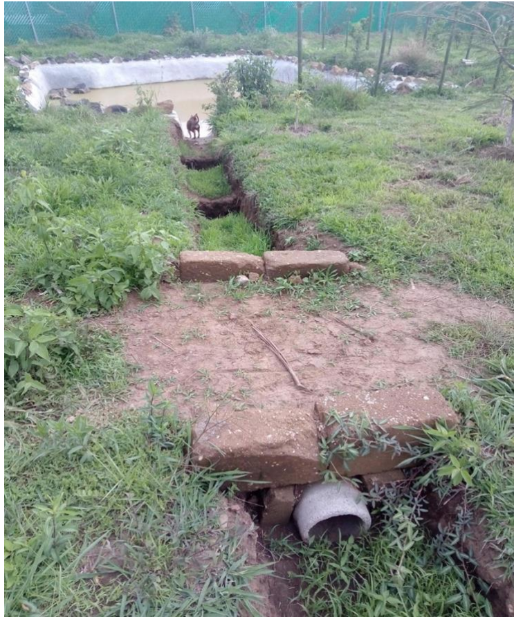
Image 4. Dried earth bricks form a small bridge over irrigation channels, which were excavated across Tierra Madre’s land to direct rainwater to a concrete storage pool. The channels did not fill with rainwater, but were often full of grasses and other young plants.
