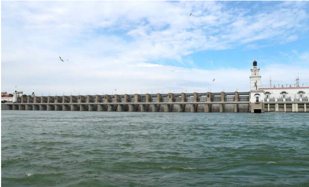
Figure 7.: Tsimlyansk Dam viewed from the downstream side (Source: imago images/ITAR-TASS)
